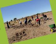
We are building the school using Hydraform blocks made of mud and concrete mix. This allows for the rapid building of the school once the foundations for each block has been laid.
